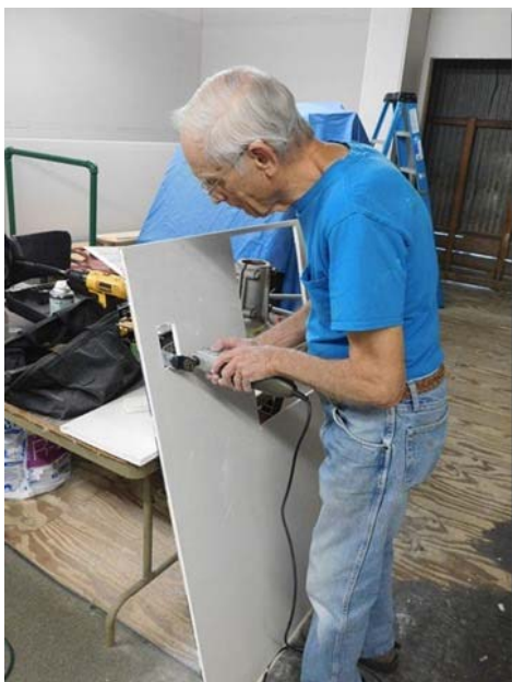
Railroad Museum Curator, Ken Murdock, works on a piece of sheetrock for the new meeting room and museum expansion area.
