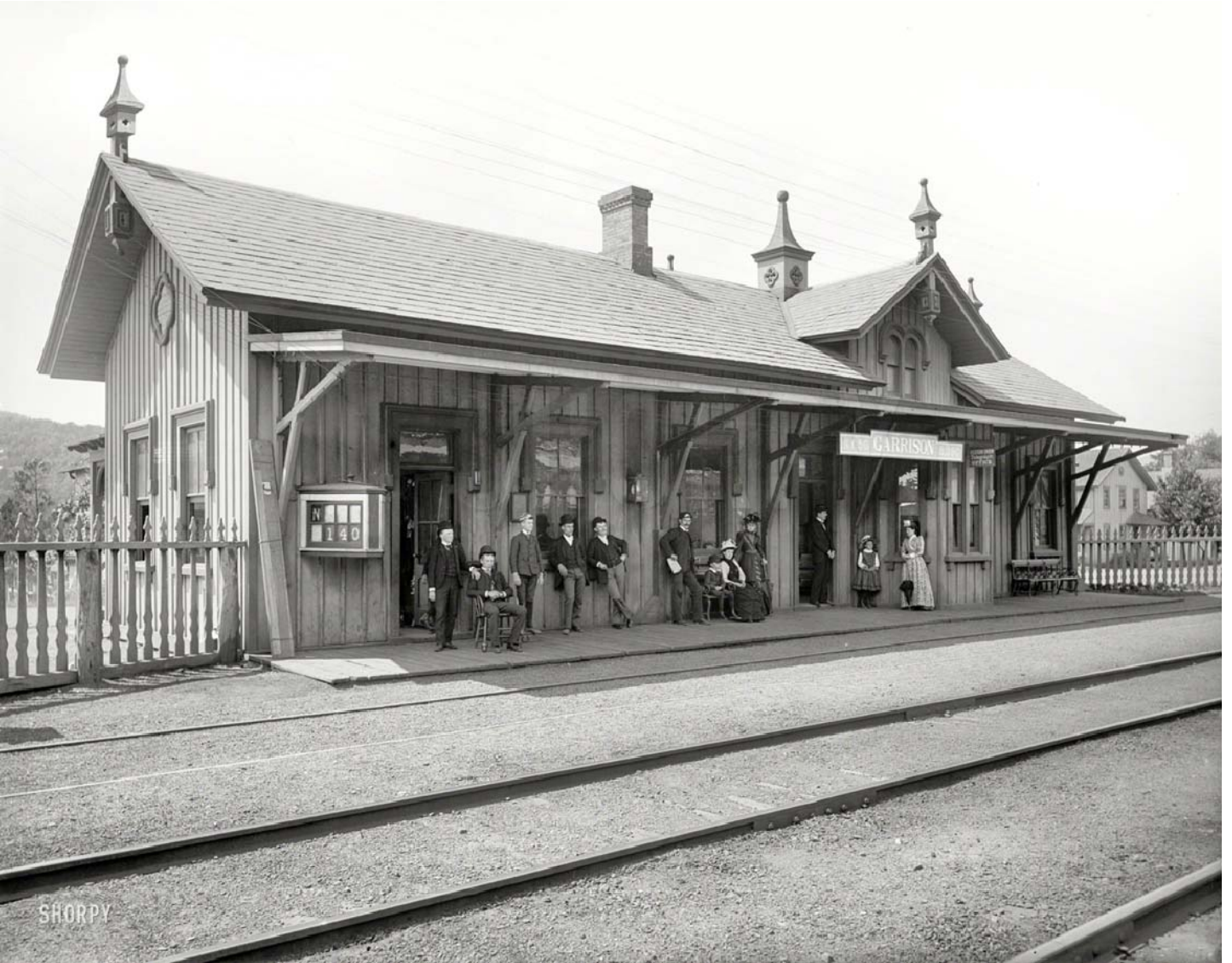
Depot at Garrison, New York, circa 1899. Garrison was on the Hudson Division of the New York Central RR, 50 miles above New York City. 8x10 glass negative, Detroit Photographic Company. Check the wire lead-ins ("drops" or "down wires") at this station. Office call sign was "GS". Photo courtesy of Society Member Warren McFarland.
