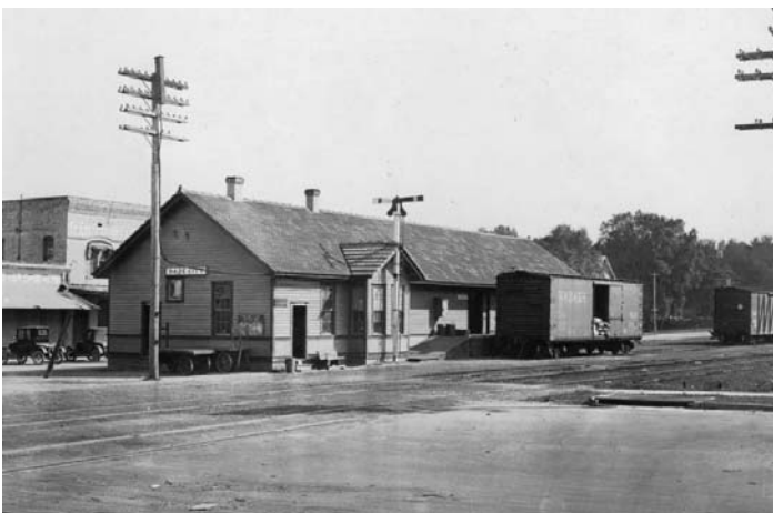
This was the Seaboard Air Line's depot in the center downtown Dade City, circa 1920. The wood frame structure was built following the standard plan for many of Seaboard's small towns, and was very similar to the one that remains in Apopka today. Irv Lipscomb photo found on Facebook
