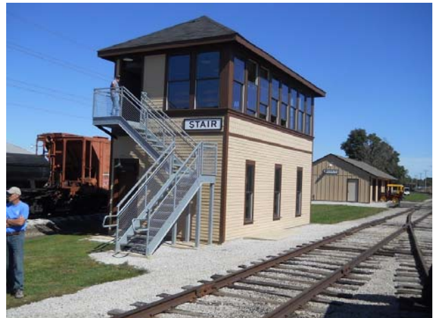
Stair Tower at the Monticello RR Museum in Illinois. It was built from Illinois Central plans and includes levers and whatnot from several demolished IC towers.
