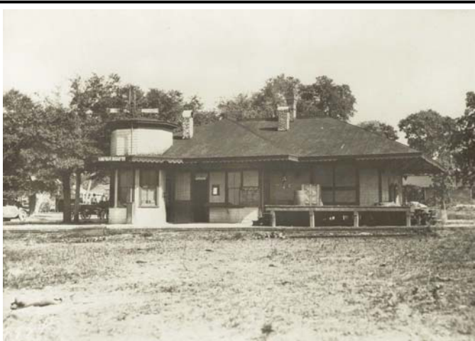
ACL Depot at Tavares, FL in 1911. Photo courtesy of Taplines.
