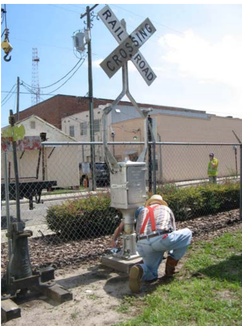
Tightening the bolts to secure the signal.
