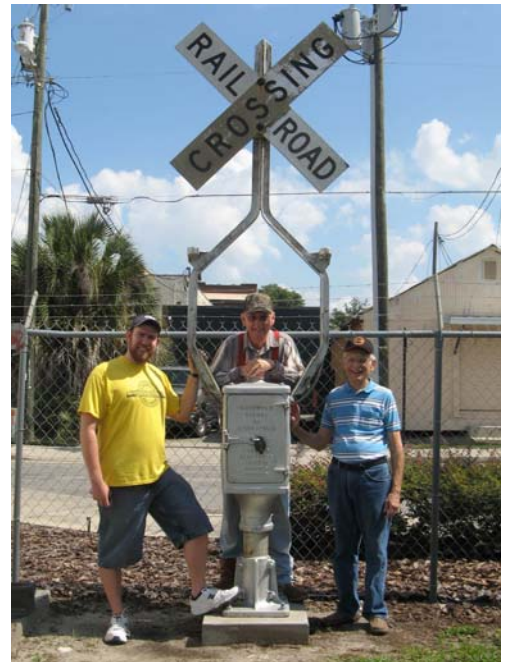
The signal installation crew.
