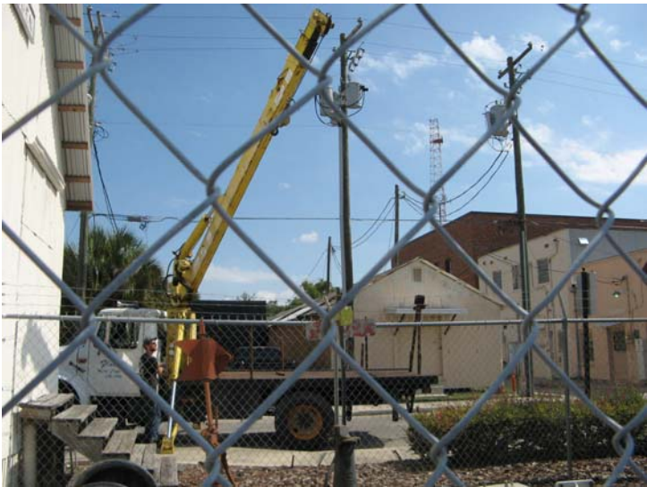
Florida Metal Craft crane truck getting ready to set the signal.
