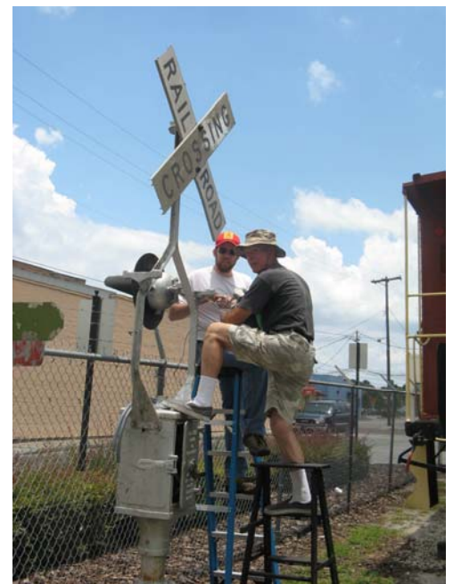
Installing the lights.
