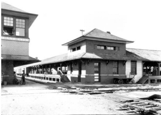
This 1924 photo shows a different tower, one that is cantilevered over the first floor walls to provide more platform space. The Plant City sign, originally recessed in the brick, no longer exists leading me to believe the tower was completely rebuilt. Another tower, built into the Railway Express freight depot, is seen across the tracks to the right. Why two towers were required remains a mystery to me. — Florida State Archives photo
