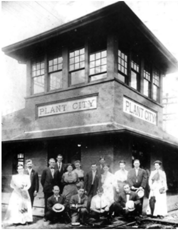
This 1911 photo shows the tower on the corner of the Plant City Union Depot which protected the diamond where SAL's main to Tampa crossed the ACL's main to Tampa. The tower brick walls, at that time, supported the tower by continuing directly to the ground below the first floor roof canopy. That arrangement left a very narrow boarding platform below the tower. — Florida State Archives photo
