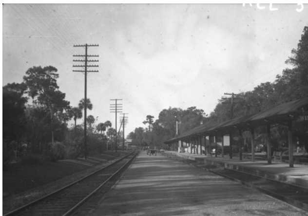
Winter Park is getting its fourth depot this year and most of us don't remember its first or second ones. This circa, 1935 photo shows their second depot, built by the ACL and located on the east side of the tracks where Morse Boulevard crosses today. The depot was accessed via a bricked cul-de-sac off of Park Avenue. - Barriger Library collection
