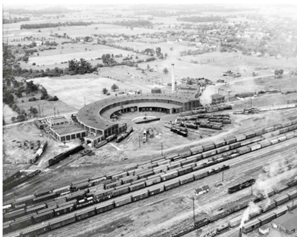
A July 1947 aerial view shows the Pennsylvania Railroad's big roundhouse at Crestline, Ohio. The long engine at middle left is No. 6100, the 6-4-4-6 duplex of 1939. Classic Trains coll.
