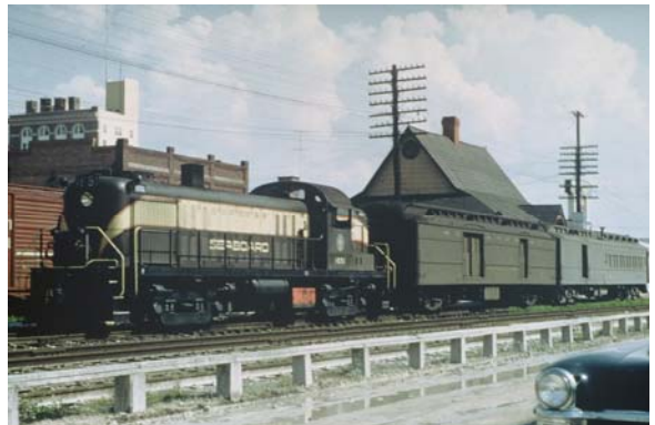
This circa 1954 scene of SAL's Orlando depot near the end of passenger service finds RS3 #1651 ready to depart for Wildwood with train #608. As it left town, it would stop at Modello Yard along U.S. 441 and pick up its freight cars. Sadly, the depot was razed in 1955 to make way for a city parking lot. - ACL & SAL HS collection
