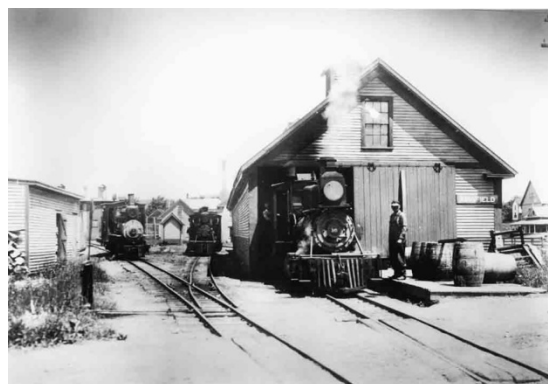
Sandy River & Rangeley Lakes 2-foot-gauge Mogul No. 16 pokes out of the covered depot at Kingfield, Maine.
